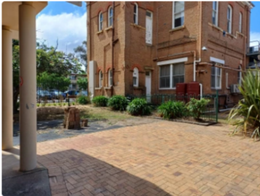
The chapel garden courtyard after the clean-up
